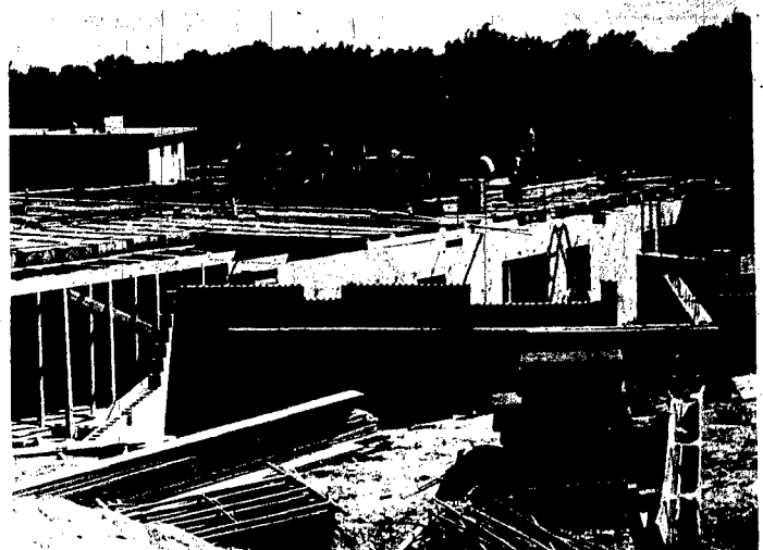
NOW A JUMBLE - SOON A CHURCH: Work is progressing fairly rapidly at the construction site of the new St. Mary's Catholic Church in Wayne. Workmen poured the first floor slab Tuesday morning and will soon begin building the frames for the concrete pillars on each corner of the six-sided building which will support the pointed roof. The contractor said Tuesday he is fairly certain the building will be enclosed by the time winter weather arrives. The new church is located to the northwest of the present St. Mary's Catholic School on East 7th St., visible in the left background.
